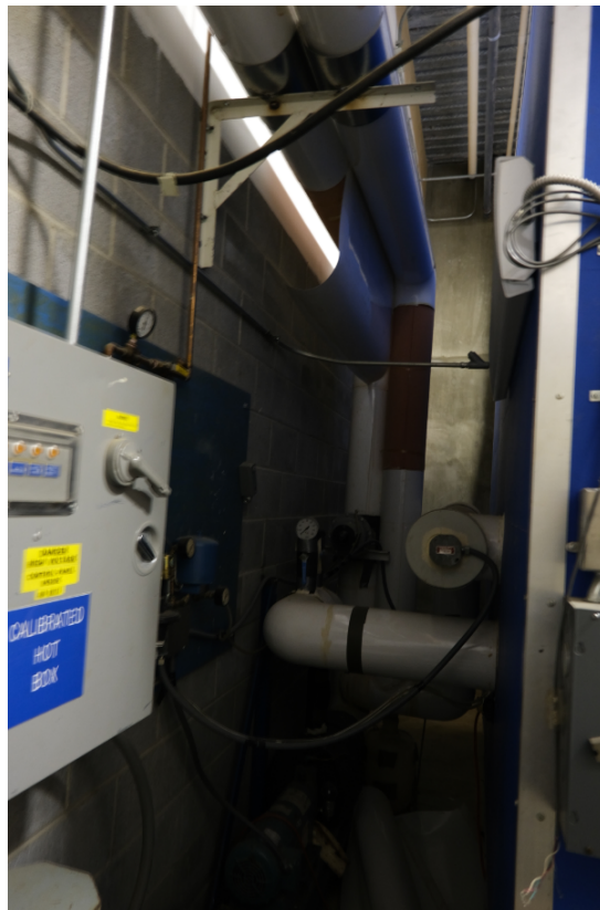
View of back of existing defunct chamber
