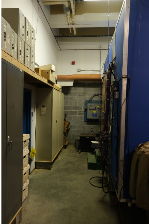
View showing limited space on left side of existing defunct chamber
