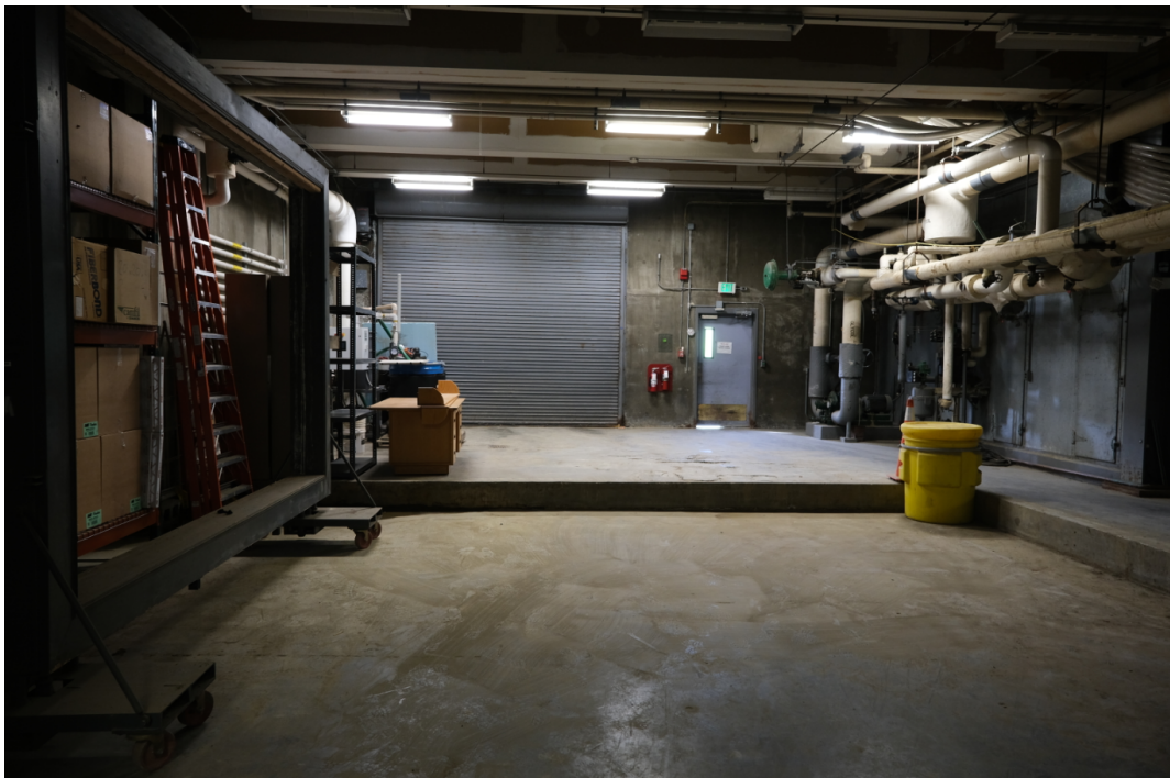
View from defunct chamber location towards exterior bay doors
