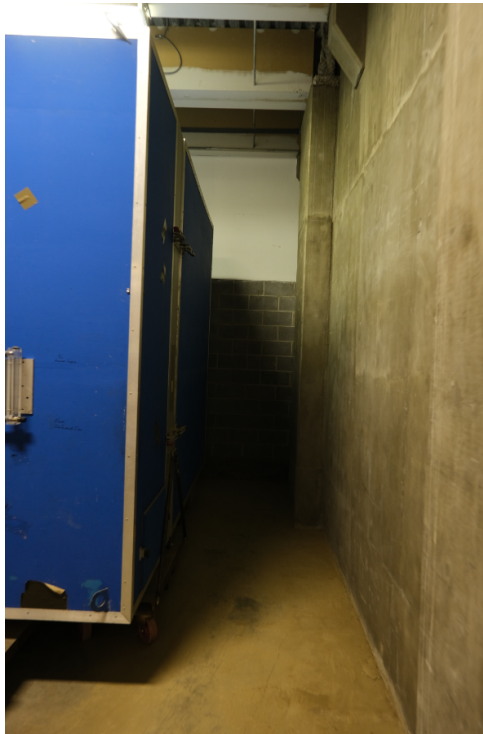
View showing limited space on right side of existing defunct chamber
