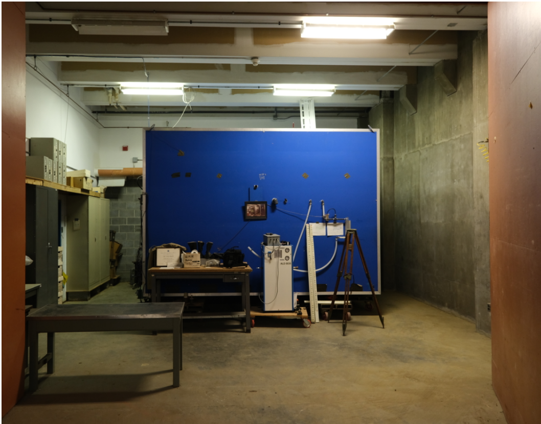
View of existing defunct chamber (will be removed/cannot be repurposed)
