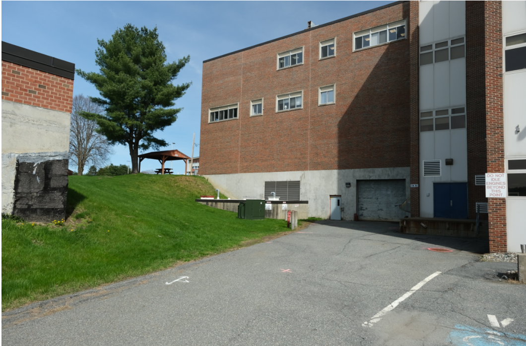
Exterior of building and bay doors into sub-basement
