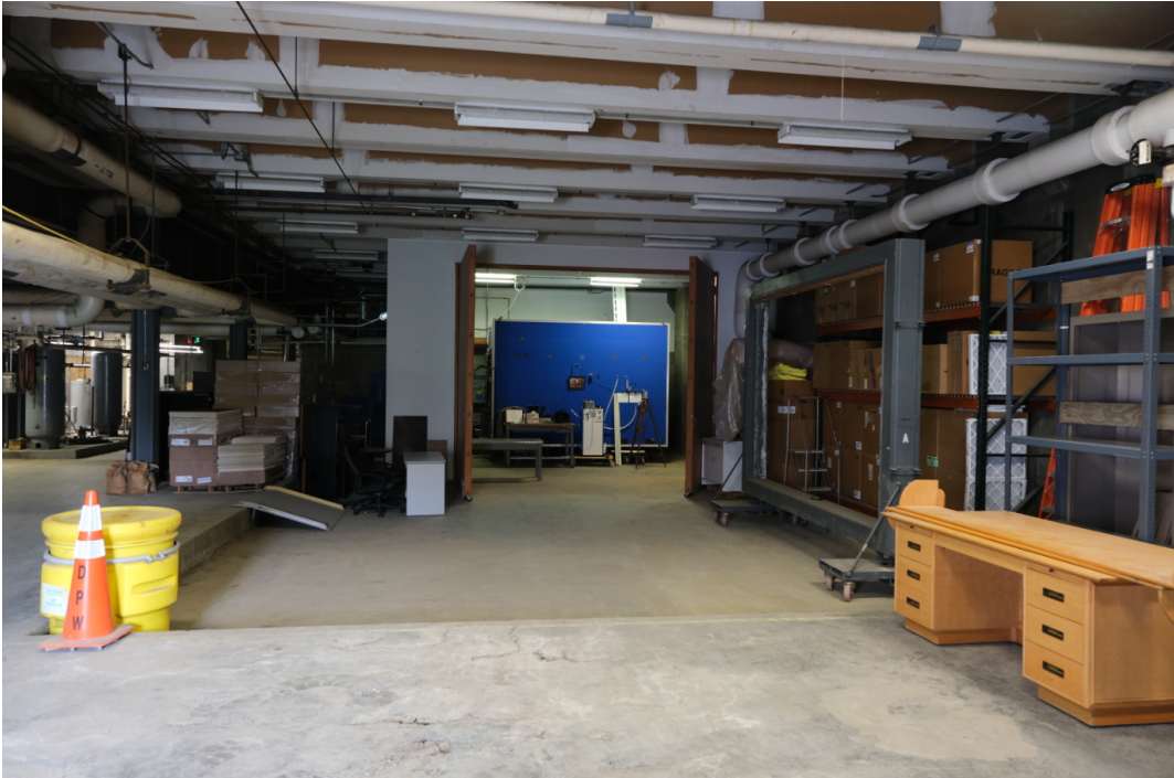
View from exterior bay doors into sub-basement
